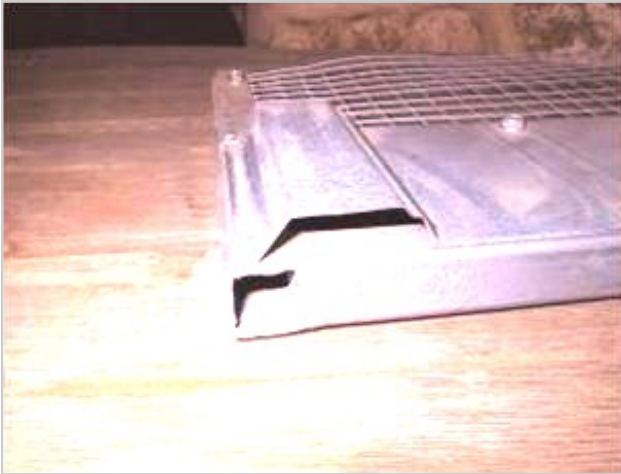
Fig. 7. Method of fixing where peak of zinalume meets edge of frame. Note also ground down weld.
